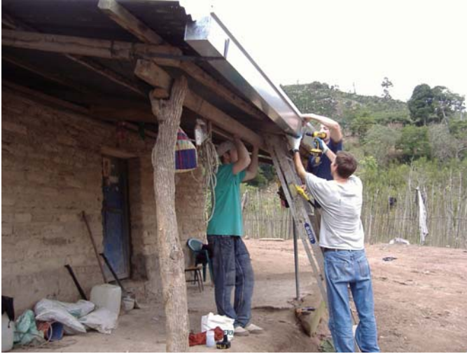
Figure 2. Students from the Student Association for International Water Issues, University of Nevada System of Higher Education, actively engaged in installing a rainwater collection system in Guatemala. Photo credit: Melanie Reed Krautstrunk.
