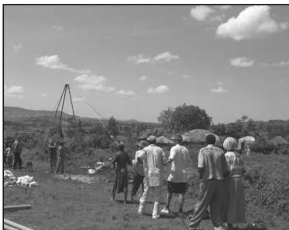
**Figure 4.** Community members and Student Association for International Water Issues volunteers drilling a water well in Rabondo, Kenya, using the reverse circulation, percussion manual well drilling method.
