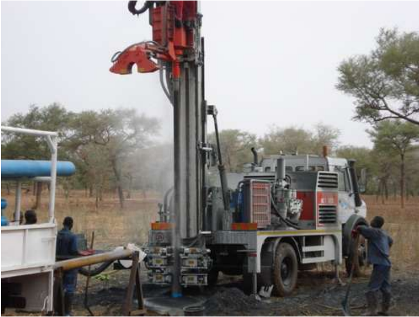
Figure 1 Drilling in Burkina Faso
